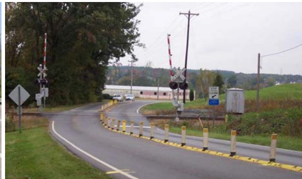
Figure 4. Gates with Channelization Devices
